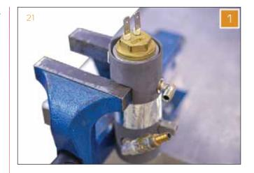
2 Using a 26 mm wrench, remove the heating element.
